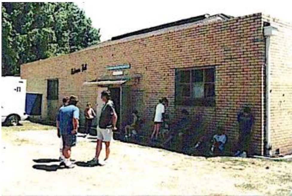
The former VAWC/VRWC clubroom, Robinson Hall on Lakeside Drive, named for Alf and Mabel – and partly built by Alf himself! (Photo: Mark Donahoo)
